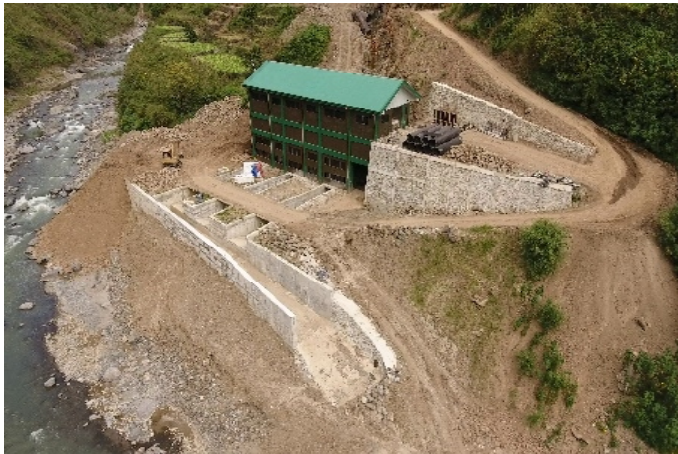
Completed Structure : (L-R) Weir, dessander and powerhouse.
