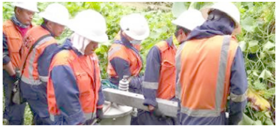
POWER RESTORATION. Linemen carefully navigates their way among vegetations carrying a distribution transformer needed for restoring power at Country Club Village, Baguio City. Beneco incurred about P12 million total cost of damages during the onslaught of Typhoons Ulysses, Ambo and Pepito last year. (CTTO)
