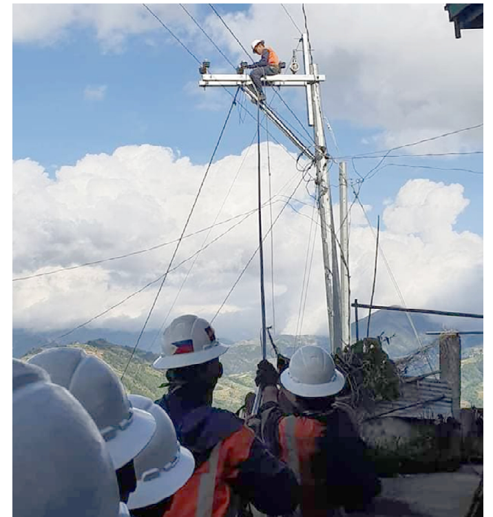
ENSURE RELIABILITY. Linemen continue to install tree wires from sitio Amgaleygey, Buguias to Sinipsip Substation as a mitigation measure to major storms and to assure the community for a reliable supply of power. (Dairic Pallogan)
